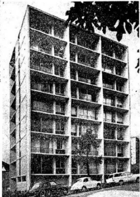
An exterior view of the new bachelor flats at Roslyn Gardens, Elizabeth Bay.
